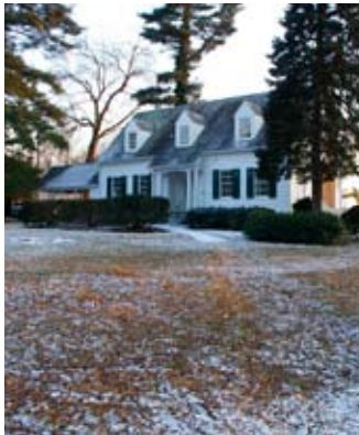
Below: The award-winning restored Frieda's Cottage.
