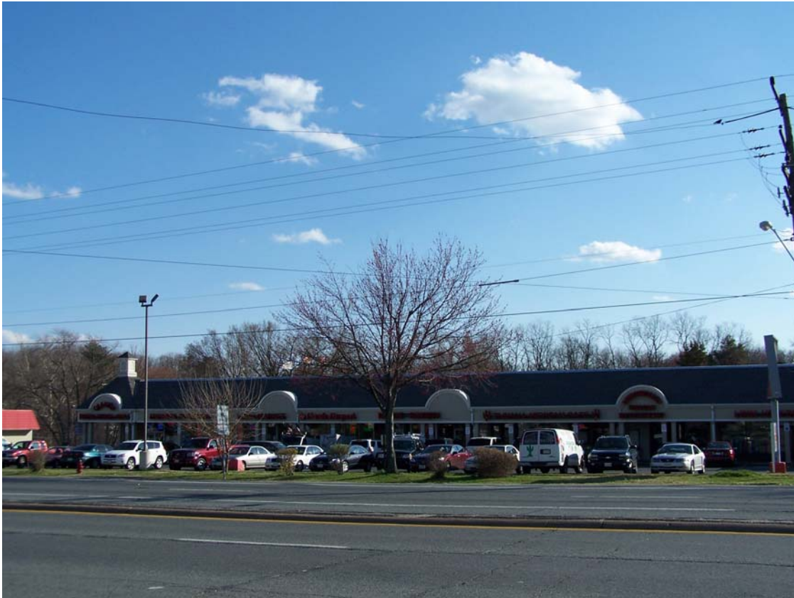
Figures 10-11. Twinbrook Shopping Mart, Rockville, Maryland; Donald Gingery, developer; façade upgraded in the 1990s (Image taken by Cindy Thompson, March 2008)
